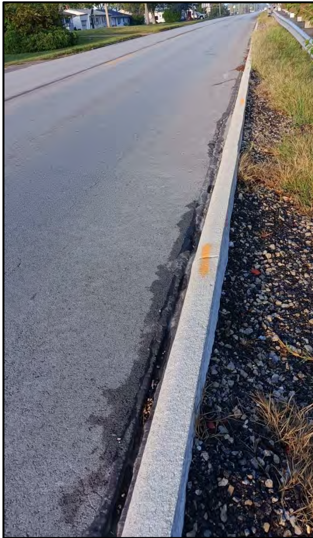
Photo 2 – Looking west, separation of curb from edge of pavement
