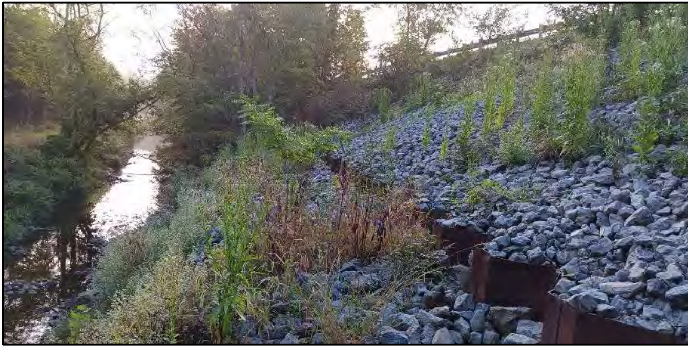
Photo 3 - Looking east near toe of slope; stream, sheet pile wall, and riprap surface
